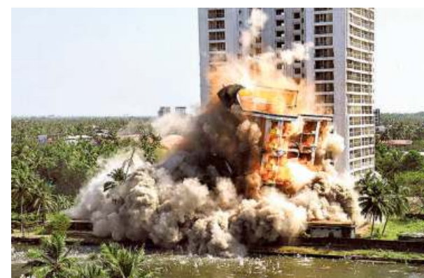
Wiped off: A view of apartments being demolished in Maradu using controlled implosion in Kochi. *FILE PHOTO
